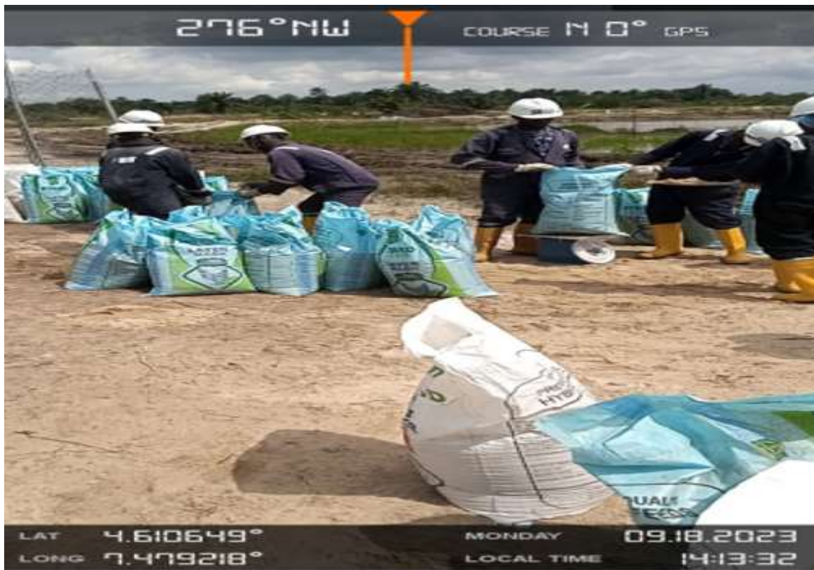
Plate 3: Sewing and Weighing of sand bags
